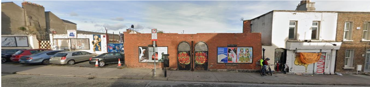
Figure 2: Street view of application site from Prussia Street
